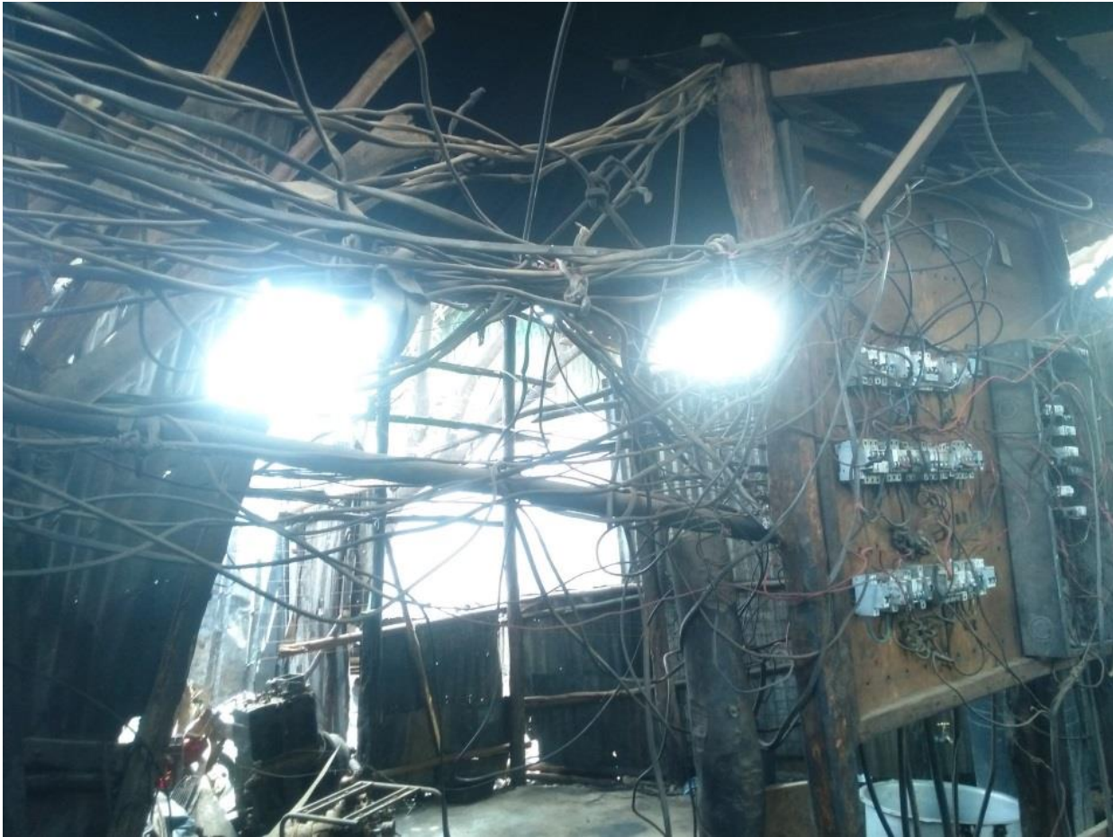
Picture: Unidentifiable where most wires start or end
