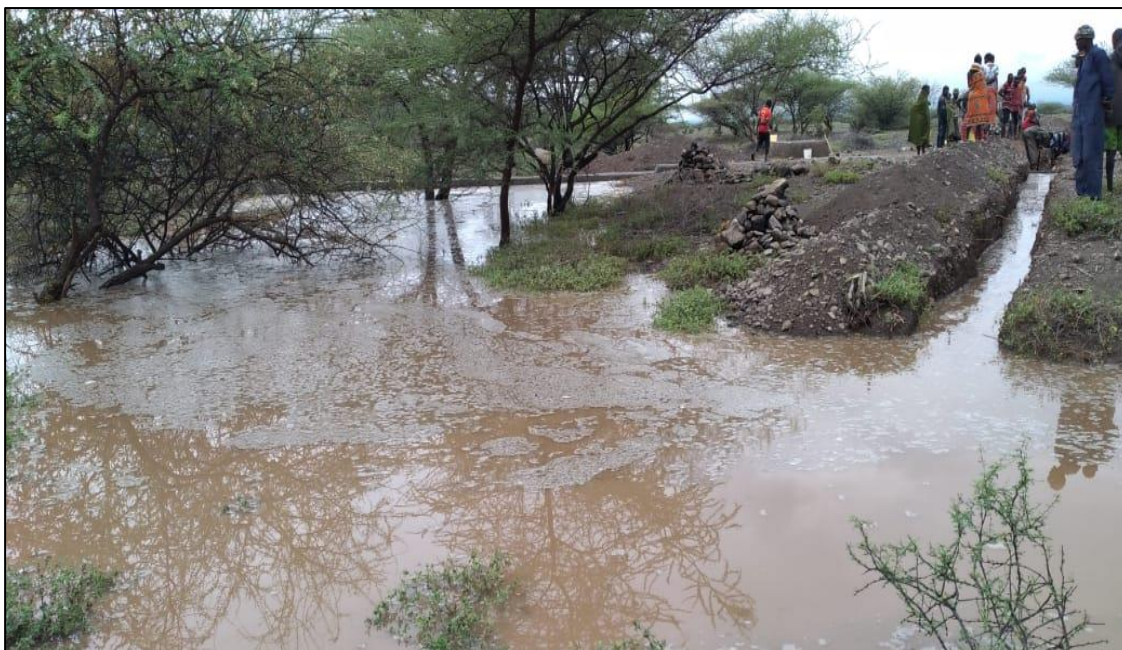
Figure 3-55: Impounded flash floods being diverted to farms
